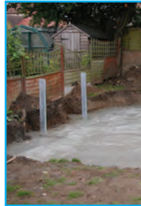
Stage 2 Lay concrete
